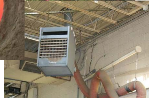
Infrared heater - Lorton, VA
