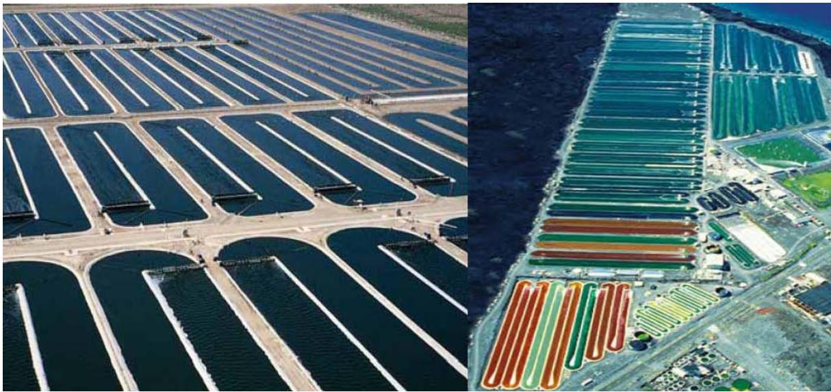
**Figure 2.1 and Figure 2.2: Commercial microalgae production in open raceway paddle-wheel mixed ponds.**
